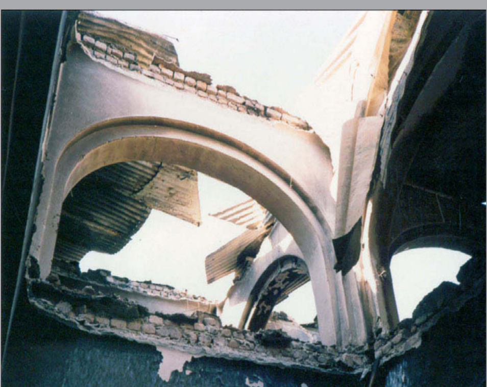
Upper floors of the National Museum after destruction in 1993.
